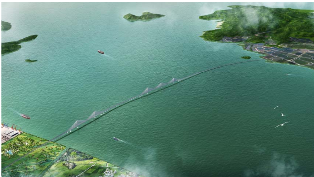
Figure 1. Overview of the Huangmaohai Link Project
