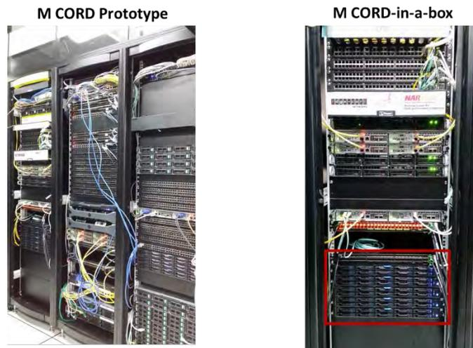
Figure 15 M-CORD-in-a-box and M CORD Prototype at NCTU
