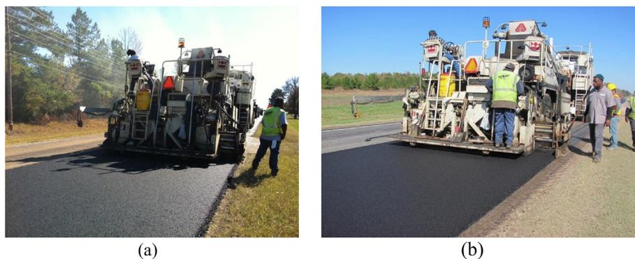
**Fig. 2.** In-situ construction environment: (a) HMA produced at 155–168 °C and (b) WMA-Evothem 3G produced at 135–143 °C (Wu et al., 2017).
