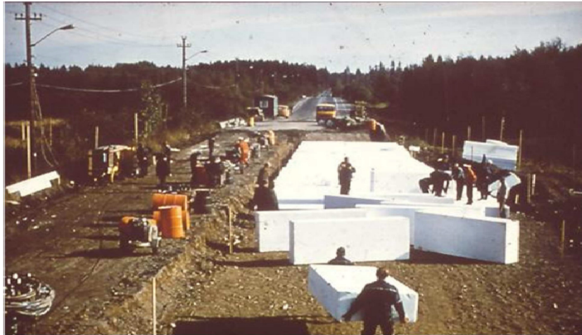
Fig. 6. EPS geofoam blocks being used as lightweight fill [27].
