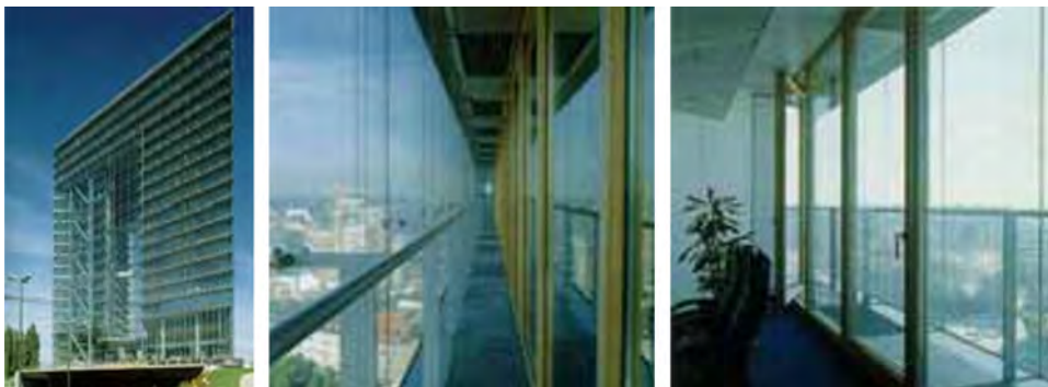
Fig. 5. Düsseldorf city gate DSF, Germany. From the left: The face; DSF cavity; Interior glazing. Source [35].
