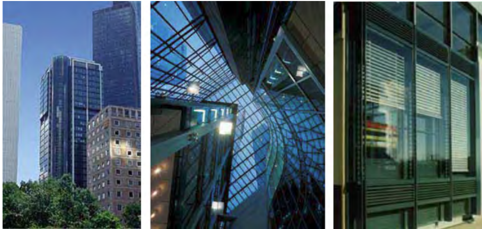
Fig. 6. Eurotheum DSF, Germany. From the left: The face; DSF interior; Shading devices. Source [35].
