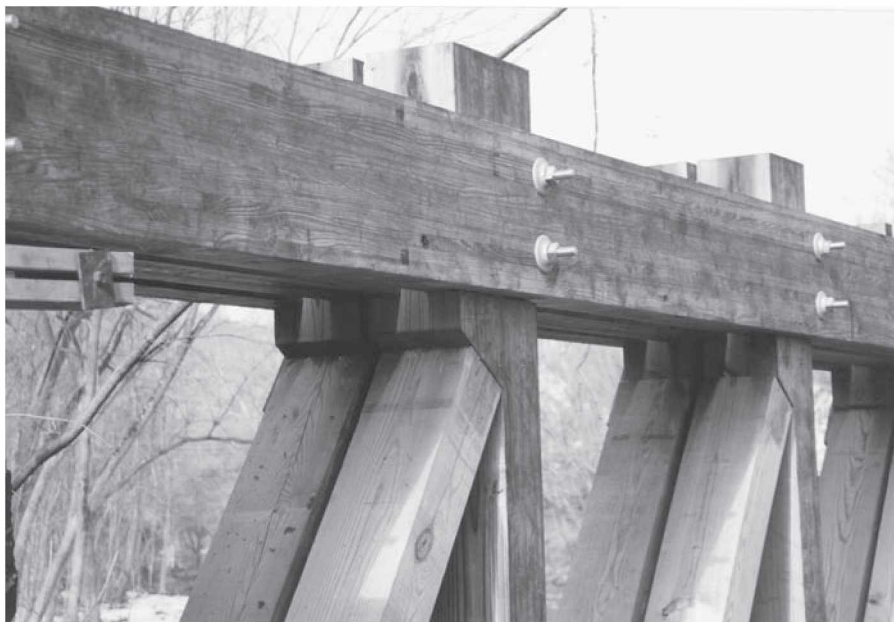
FIGURE 18-4 The chords are pressure-treated glued laminated timber.
