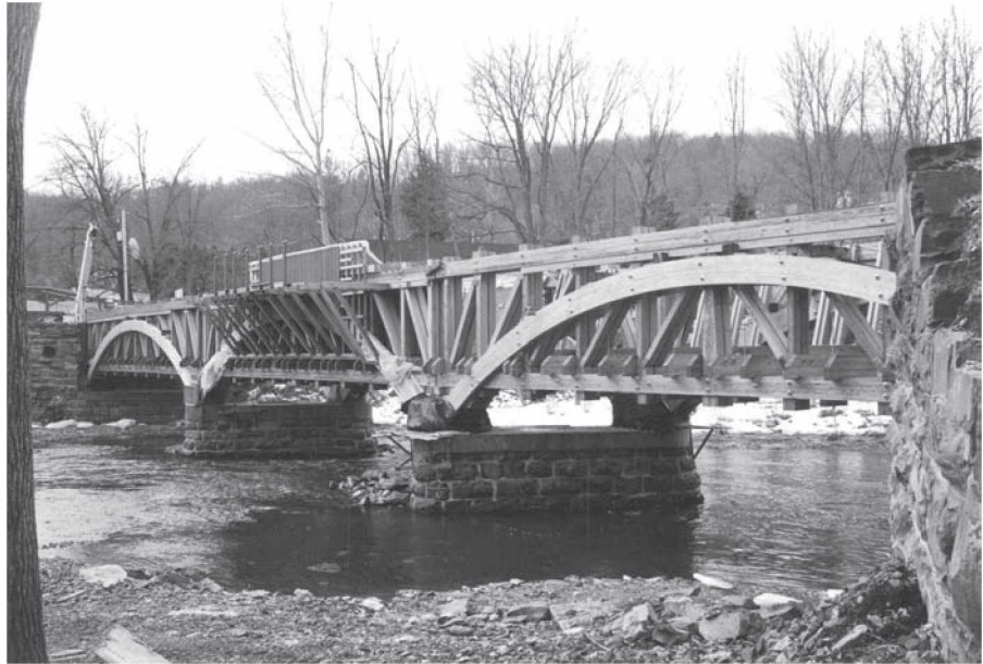
FIGURE 18-1 The aqueduct consists of three equal spans of 66 feet. (See color insert.)
