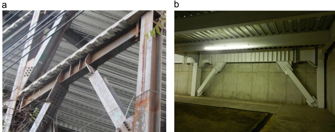
Fig. 1. Examples of the use of eccentric braced frames in buildings: a) short link, b) long link.
