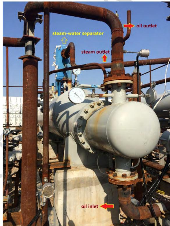
Fig. 5. Photograph of the evaporator.
