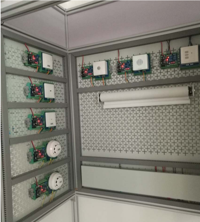
Fig.4. Information domestic appliance R&D center
