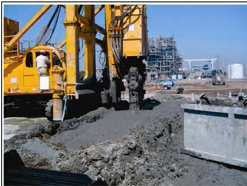
**Figure 6b. TRD milling wall.**
