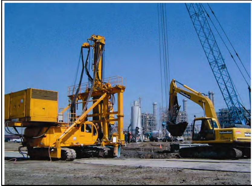
**Figure 6a. TRD milling wall, and excavator removing spoils**
