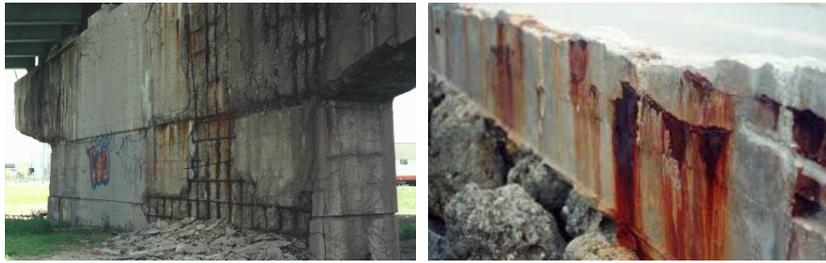
Fig. 8. Reinforcement corrosion of the structure parts in contact with soil.
