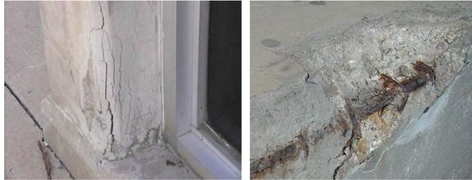
Fig. 5. Concrete carbonation paved the way for frost action.
