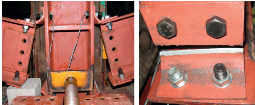
(a) Failed connection
