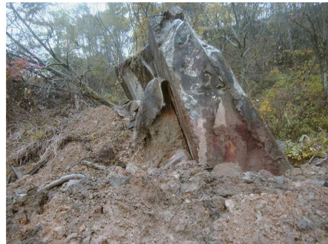
Fig. 2. Gravity retaining wall in Takamachi-danchi residential area damaged during the October 23, 2004 Chuetsu earthquake, Niigata, Japan.
