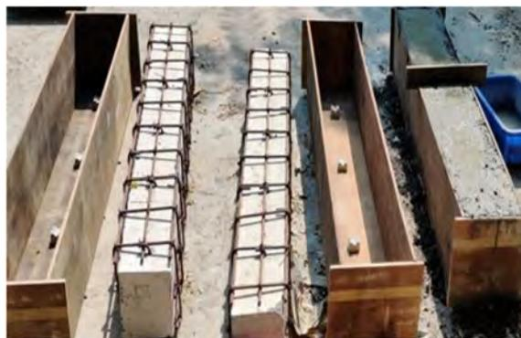
Fig. 6. Concrete jacketing process in columns with wooden moulds.
