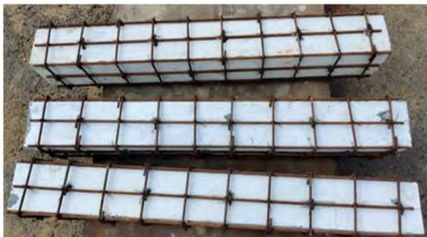
Fig. 5. Strengthening with steel reinforcement.
