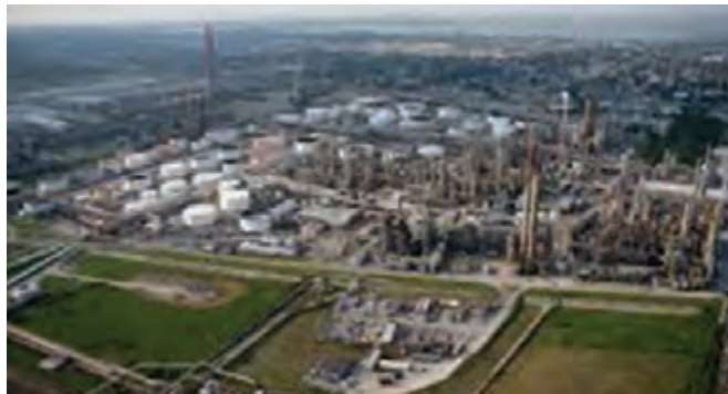
Fig.9: A chemical plant
