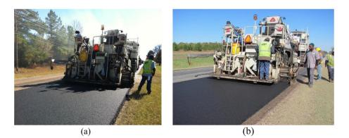
Fig. 2. In-situ construction environment: (a) HMA produced at 155–168 °C and (b) WMA-Evotherm 3G produced at 135–143 °C (Wu et al., 2017).
