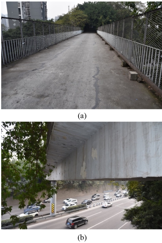
Fig. 3. Test bridge: (a) pavement surface; (b) side view and underneath traffic.
