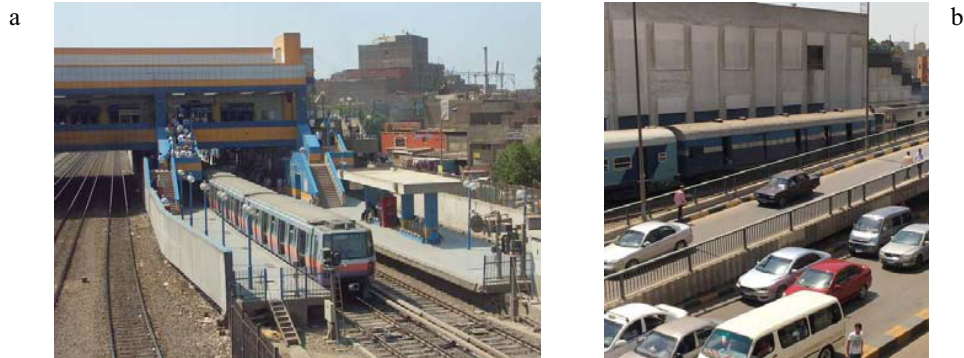
Fig. 5. (a) Shows the metro station , (b) shows Saft el laban corridor
