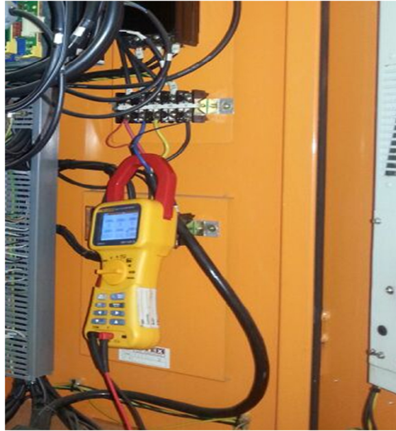
Figure.1. Photograph of the power quality analyzer connected to the CNC machine
