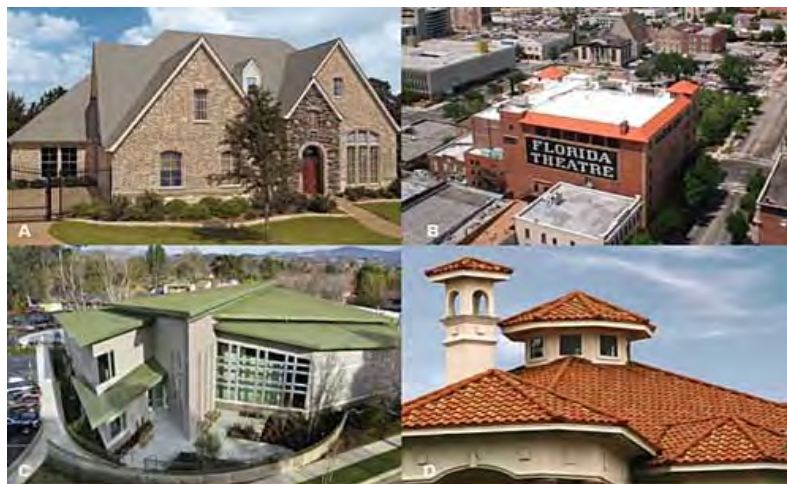
Figure 4: different roofs using cool roofing materials (such as clay and metal covers) to have maximum sunlight reflection.
