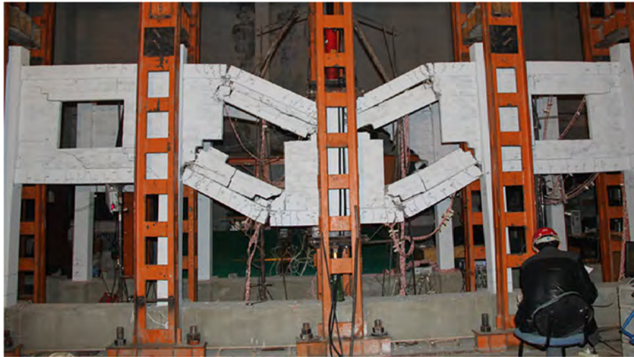
Fig. 12. Test by Shan et al. [198] on an RC frame with infill walls. Photo by courtesy of Shuang Li (Harbin Institute of Technology).
