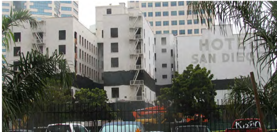
Fig. 16. Hotel San Diego used for testing by Sasani and Sagioglu [218] and Sasani [219]. Photo by courtesy of Mehrdad Sasani (Northeastern University).
