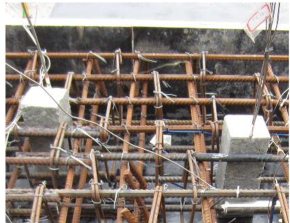
Fig. 10. Precast concrete blocks with thermal couples.
