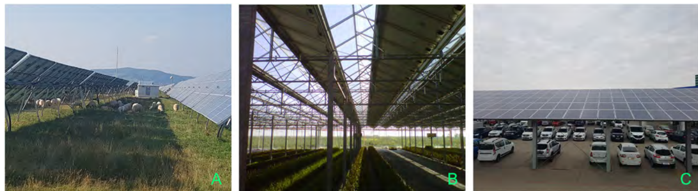
Fig. 17. Examples of types of land used to install PV power plants on, where the land has practical outcomes (Panel A – grassland for animals (Ucea de Sus, Romania), Panel B – greenhouse for various plants, Panel C –PV solar parking lot (Bucharest, Romania)).
