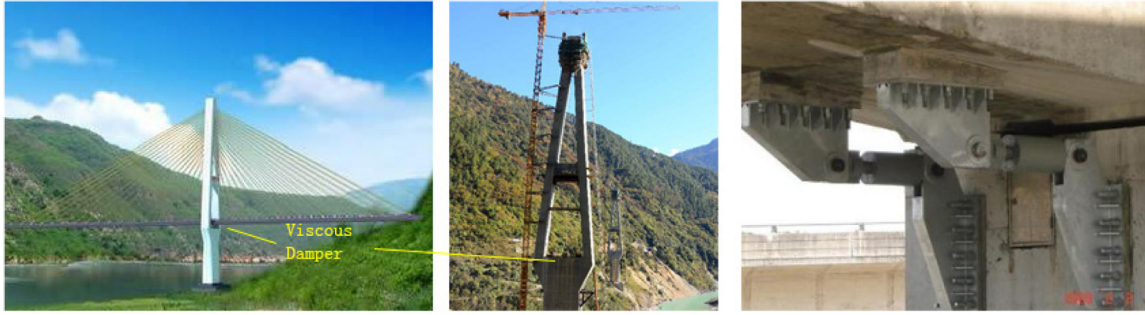
Figure 6. The Polonggou Bridge during construction and the application of FVD.
