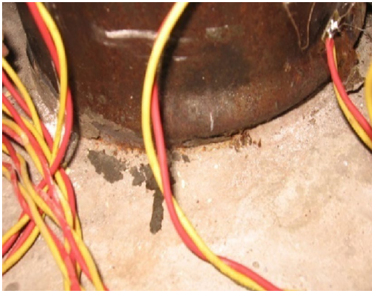
Fig. 4 Failure mode of specimen
