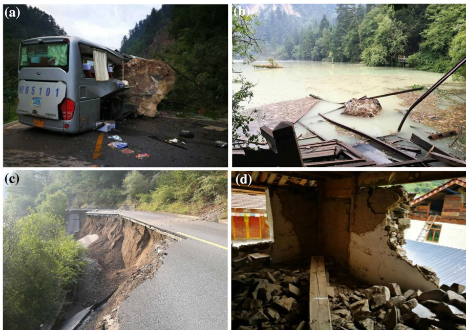
Fig. 4 Maps of damages after Jiuzhaigou earthquake. a Bus damaged by falling rocks; b infrastructure damage in scenic spot; c road collapse; d house damage. Sources: http://www.xinhuanet.com/ , http://www.chinanews.com/ and China Earthquake Administration http://www.cea.gov.cn/
