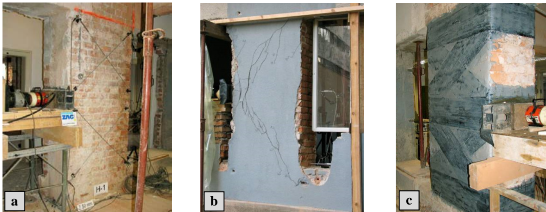
Fig. 2. Test setup on wall H1 (a), shear damage of wall H2 (b) and strengthened wall H1 (c).
