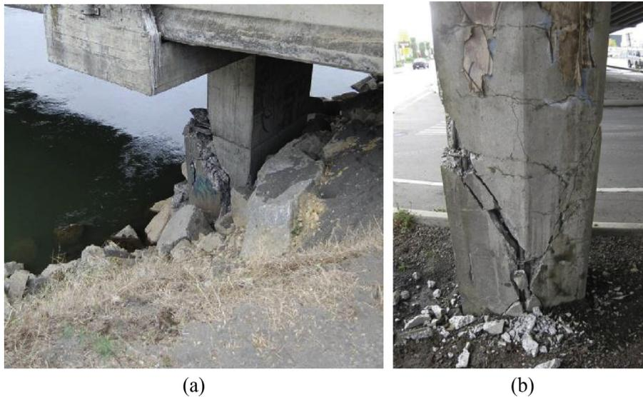
**Fig. 1.** Typical damage experienced by existing reinforced concrete bridges after an earthquake: detail of shear failure at the pier base, (a) Juan Pablo II Bridge affected by 2010 Chile Earthquake [72], (b) Moorhouse Avenue Overbridge affected by 2011 Christchurch earthquake [74].
