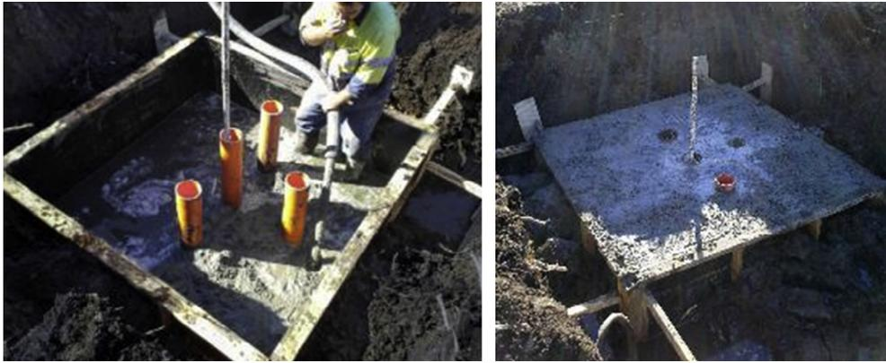
**Fig. 7.** Foundation construction (left) Pouring concrete into foundation formwork around instrumentation tubes (right) completed foundation after casting.
