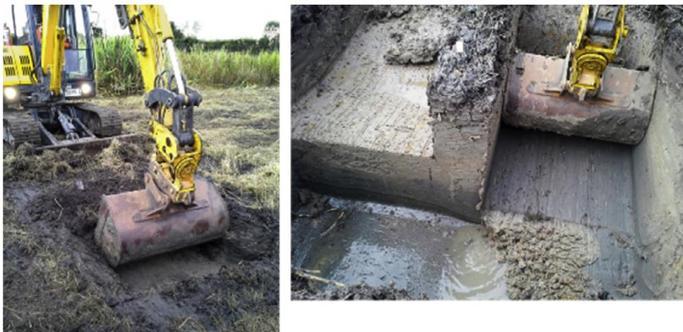
Fig. 6. Foundation excavation indicating free-standing vertical trench walls.
