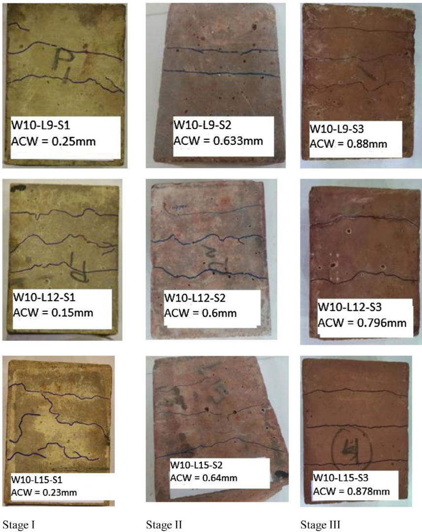
Figure 6. Crack pattern of reinforced concrete blocks prepared with reinforcing steel spaced at 30–50 mm and subjected to three different levels of corrosion treatment.
