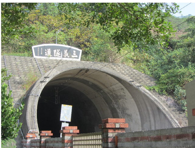
Fig. 2. Sanyi tunnel (SSR200 2013).
