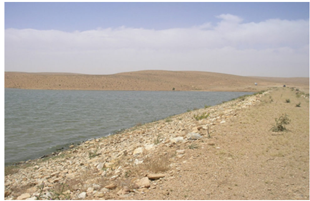
Fig. 1 View of the dam
