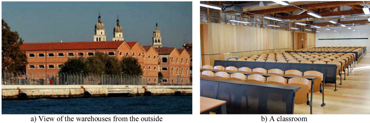
Fig. 2. Views of the warehouses.
