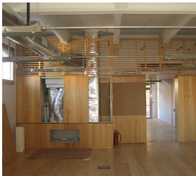
a) AHU partly covered
