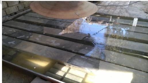
Figure (5): Curing of Spliced Reinforced Concrete Girders
