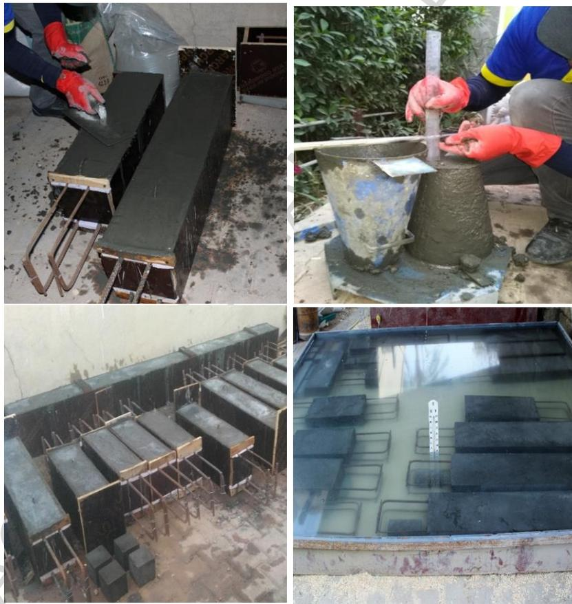
Figure (3): The Stages of Casting and Curing of Precast Concrete Segments
