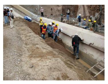
Figure 10: Distributed temperature sensing cable installation at plinth level
