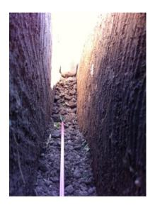
Figure 15: Installation of SMART profile sensor in a trench on the protected side of the levee
