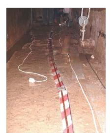
Figure 14: Installation of SmarTape and Temperature Sensing Cable
