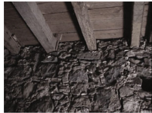
Fig. 7 Type A (a) and Type B (b) stone masonry walls fabric and arrangement
