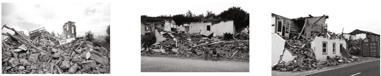
Fig. 1 Severe damage recorded in Faial island after the 1998 Azores earthquake
