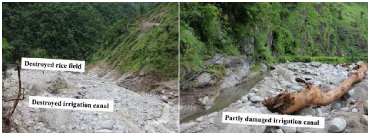
Fig. 4 Damage to the irrigation canals due to 2017 flash flood
