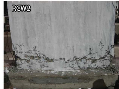
Cracks concentrates at the bottom
