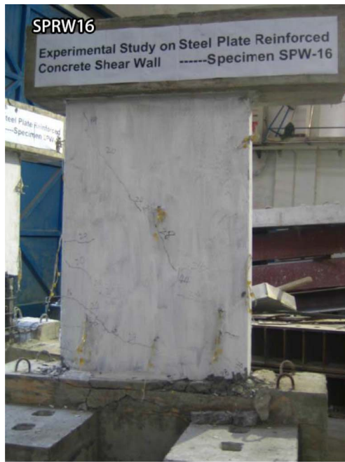
Crack between bottom beam and wall
