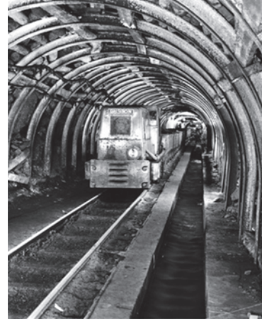
FIGURE 2: The haulage roadway.
