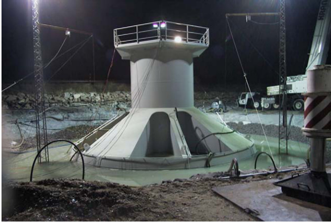
Fig. 1. Bucket foundation after installation in Nov., 2002.
