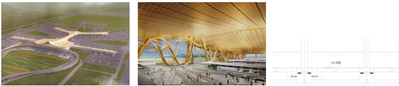
Fig. 14 Seismic Isolation of new Kunming airport Terminal (2007-2012)
