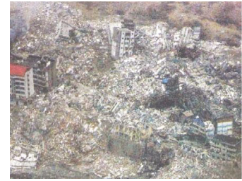
Fig. 3 Buildings collapsed in Wenchuan
