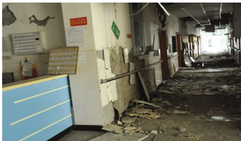
Fig. 5 Two buildings without isolation in Lushan County Hospital, damaged
