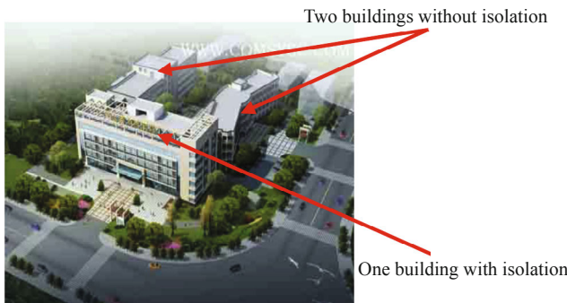
Fig. 4 Lushan County Hospital, including three buildings
