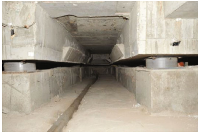
Fig. 18 Base Isolation retrofit in Shaanxi Province
