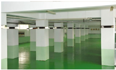
Fig. 19 1st story isolation retrofit in Shaanxi Province
