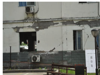
Fig. 5 Two buildings without isolation in Lushan County Hospital, damaged
