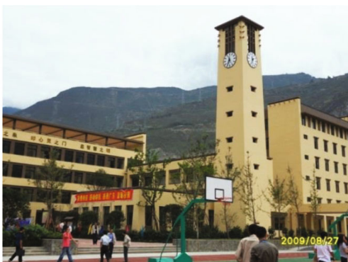
Fig. 11 Seismically Isolated building school in Wenchuan County
