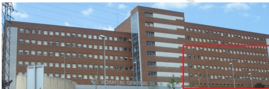
Figure 1: Hospital section where the monitoring system was installed.
