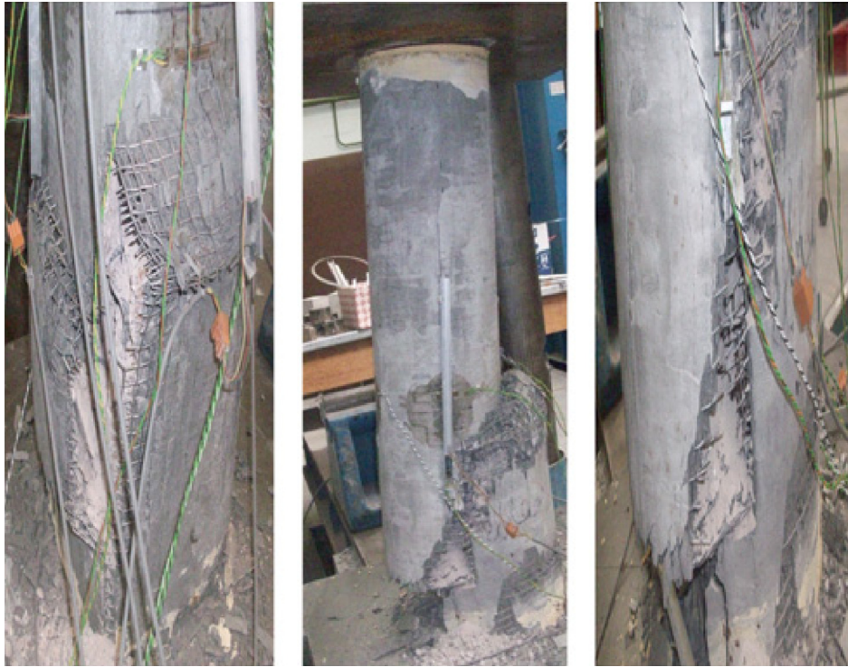
Fig. 6. Crack pattern of ferrocement jacketed circular columns [15].
