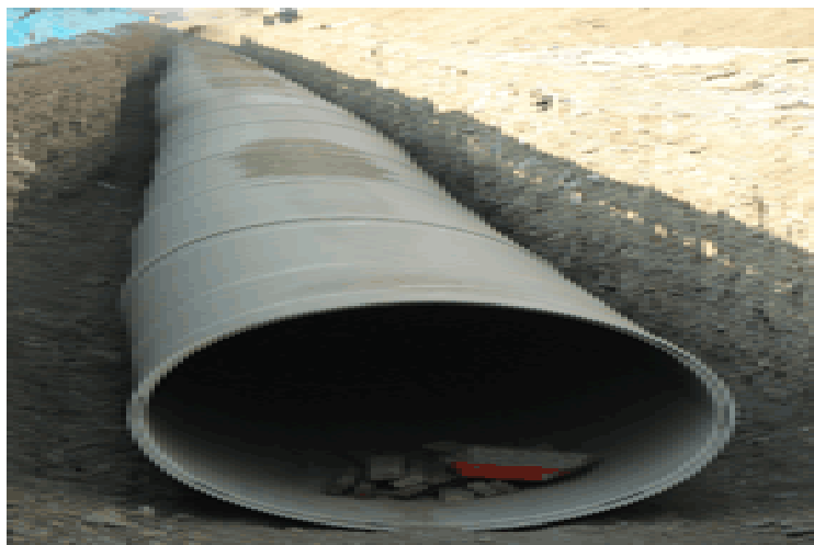
Figure 2. Urban utility tunnel district 22 of Tehran.
