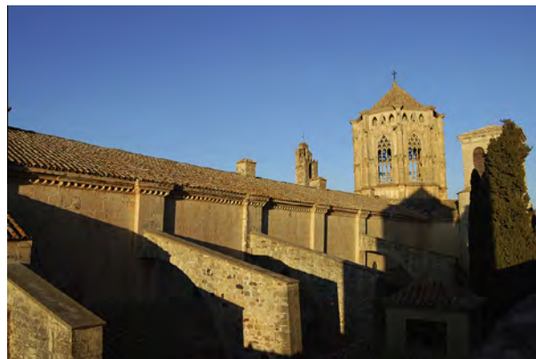
Fig. 6. The three flying buttresses at the southern part of the church constructed during the restoration of the 19th century.
