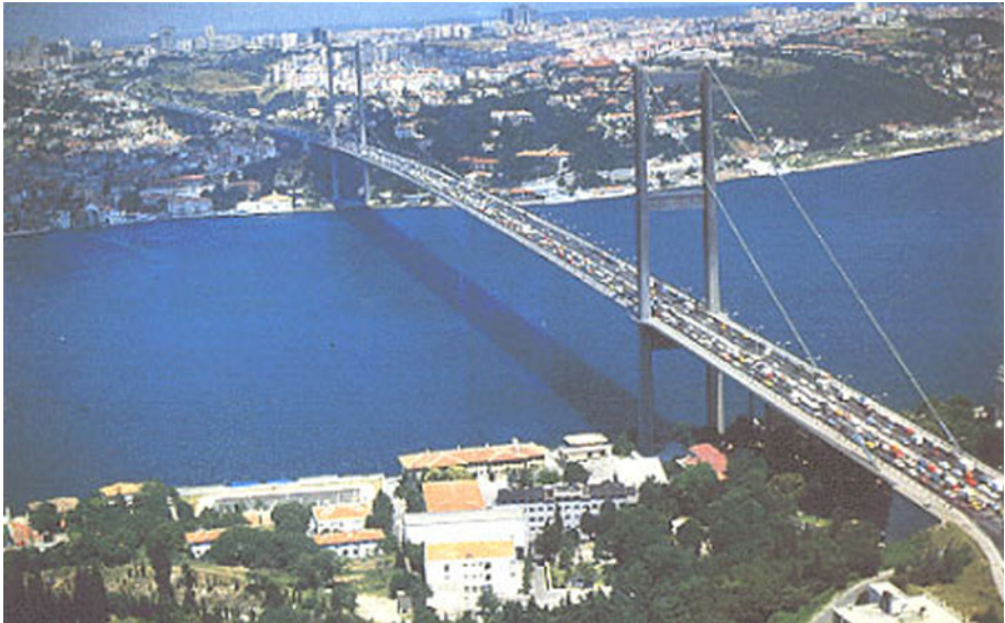
Fig. 5 Picture of Boğaziçi (First Bosphorus) Suspension Bridge ( http://www.oib.gov.tr/portfoy/bogazici_koprusu.htm )
