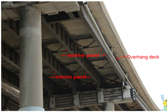
Fig. 1. Overhang deck in a typical steel girder bridge.
