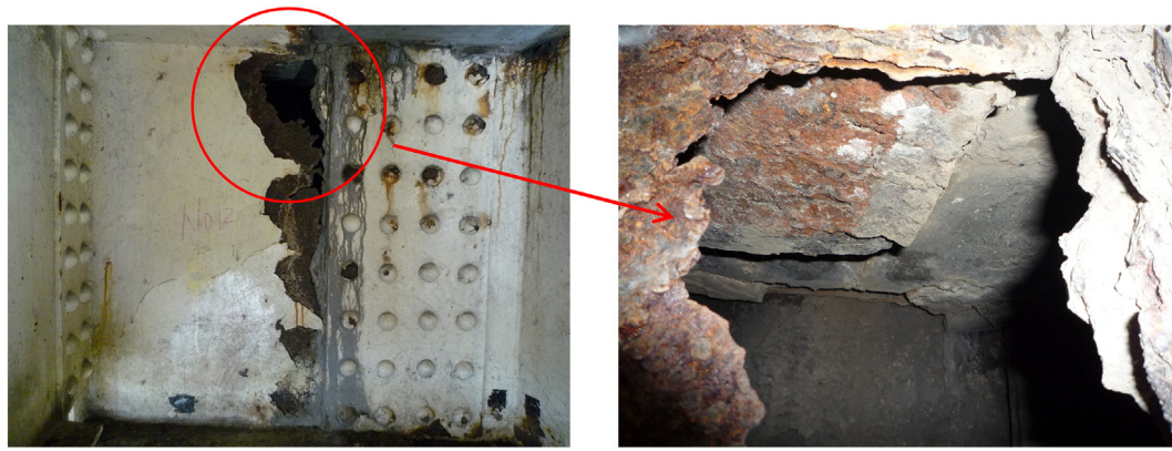
Fig. 1. End cross-girder.
