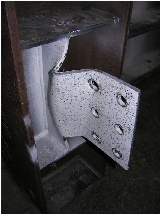
Fig. 8. Out-of-plane Deformation of Stabilized Specimen.
