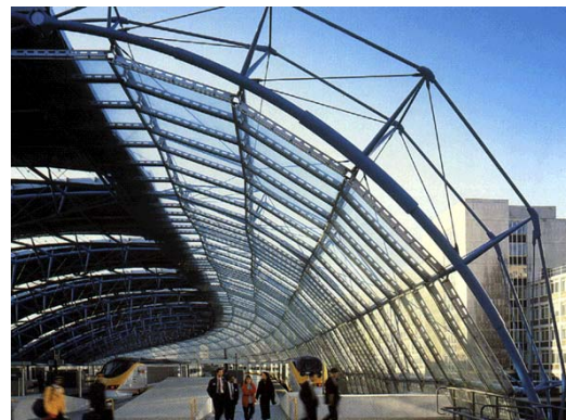
Figure 3. The interior view showing bowstring-shaped steel trusses of Waterloo International Terminal.
