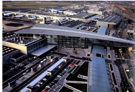
Figure 6. The exterior view of the terminal 3 and the train station, Copenhagen Airport, Denmark.
